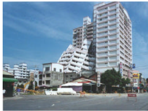
Photo 4 Collapse of a high-rise apartment building in Dali
