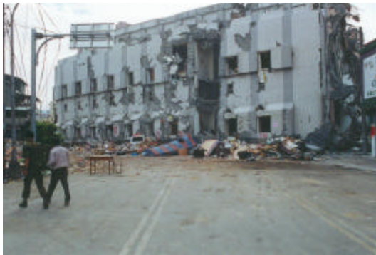
Photo 3 Collapse of a apartment building in Fengyuan
