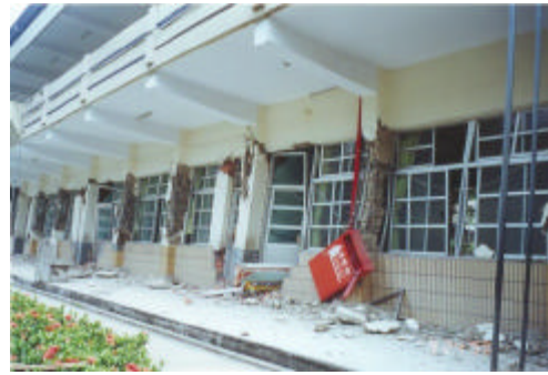
Photo 2 Shear failure of RC columns due to the short column effect
