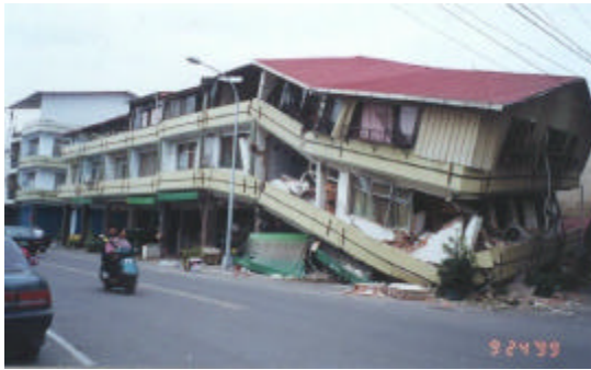
Photo 1 Collapse of the typical building having pedestrian corridor
